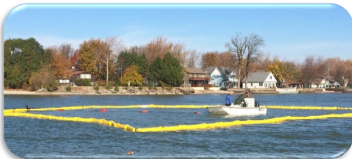
Zequanox is applied to the treatment area by PLM crews via specialized injection system.
